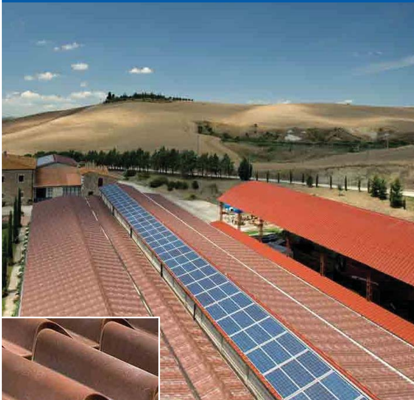
Renovation of an agricultural building in Pienza
