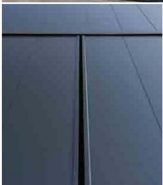
Detail of the work
