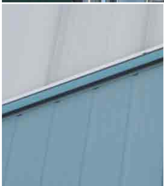
Detail of the wall
