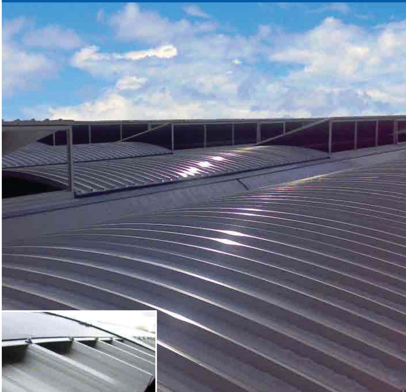
Industrial roof on a prefabricated concrete building
