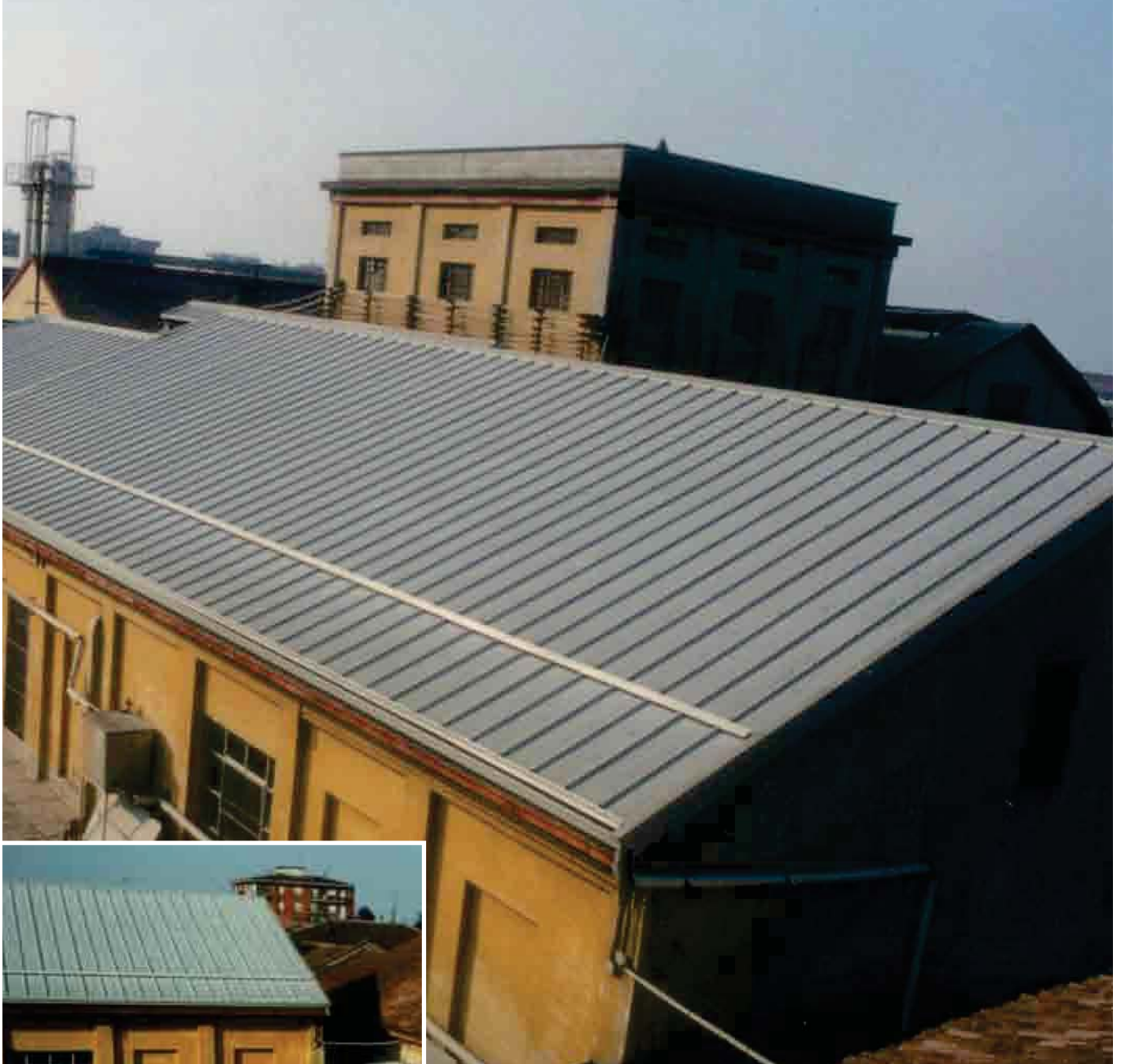
Roof of a dairy centre in Cremona
